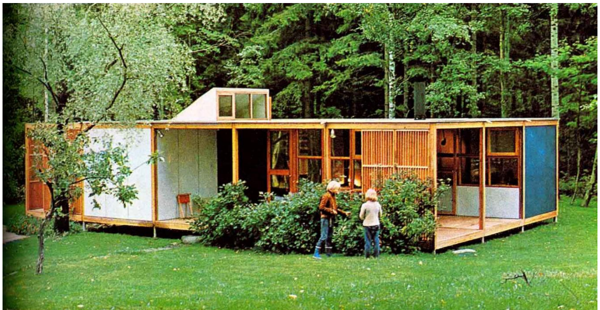
Fig. 2. Residential unit Moduli 225, Helsinki. This project for a summer home designed by Kristian Gullichsen and Juhani Pallasmaa in 1971 was considered an effort to enhance the corporeal relationship between people and nature. Source: Eba, 2013
